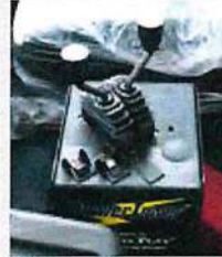
Inside air controls in power tower
